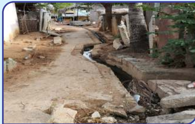
Drainage system half done and blocked.
