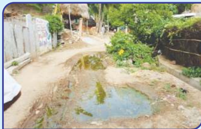
Lack of hygiene because of improper liquid waste disposal system & rain water harvesting mechanisms.
