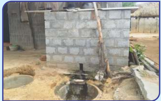
Half-done toilets with drainage exposed spreading diseases.
