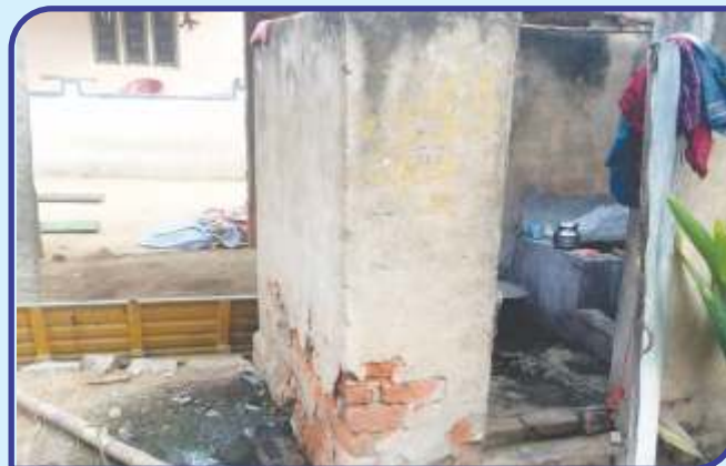
Toilets without water supply, proper drainage & Doors making them unusable.
